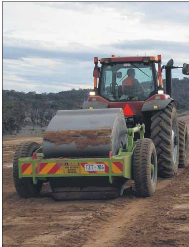
Compaction: With just six to 10 passes of the Broons' impact roller applied of surface, improvement in density can occur to at least 1m.
