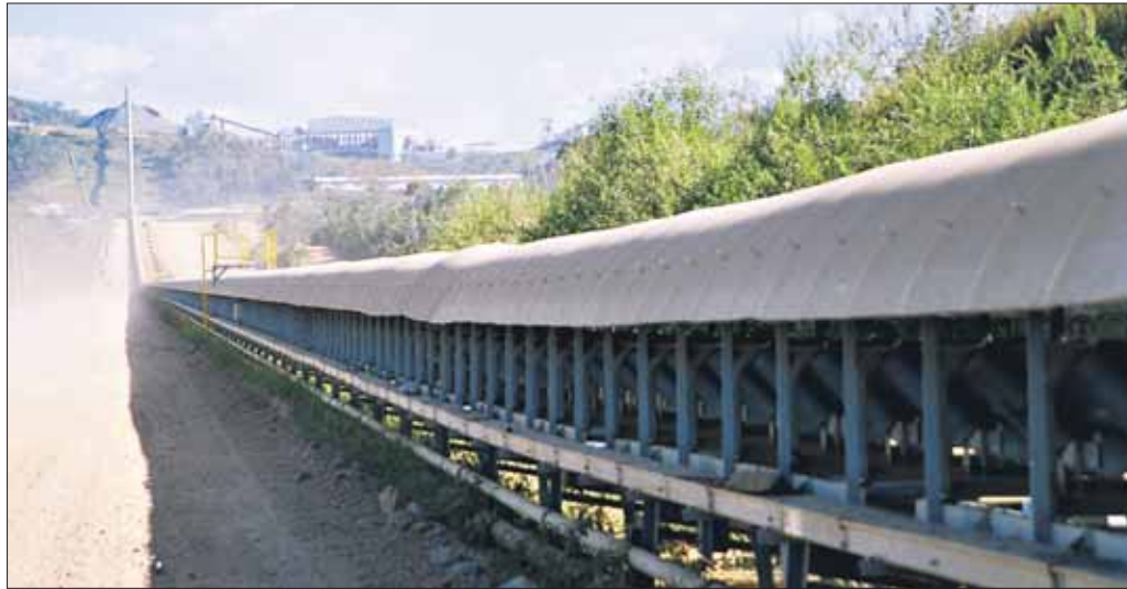
Expansion: Under the terms of a multi-million dollar agreement, Swiss-based technology giant ABB will supply electrical and automation systems at Vale's S11D iron ore project in northern Brazil.
